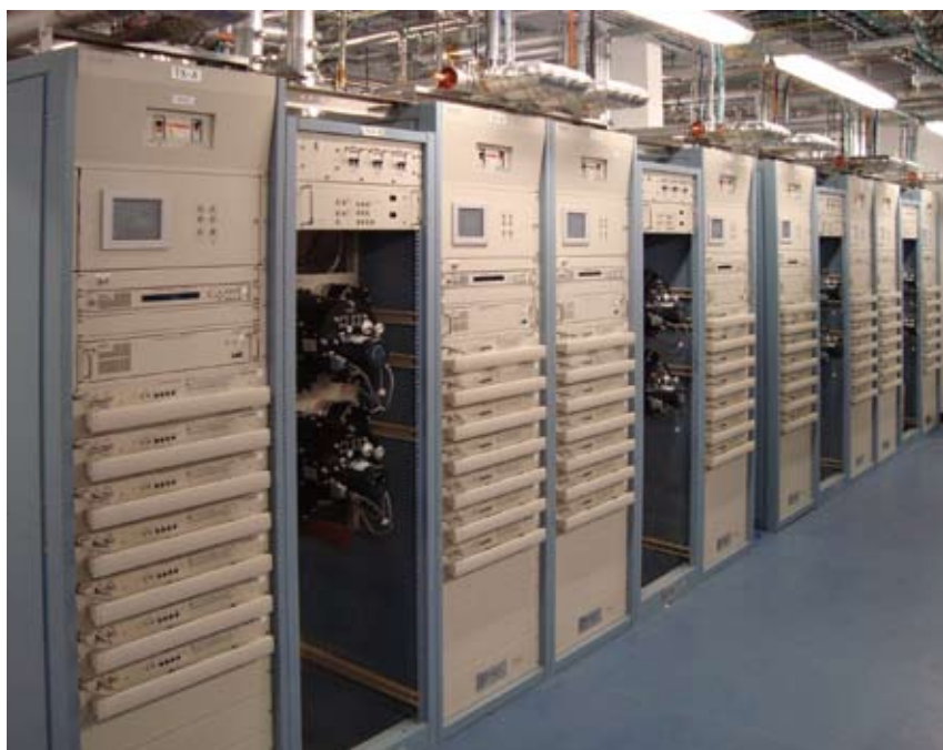
A DVB-T2 compliant DTU-52 Series installed at Winter Hill (U.K.) for Arqiva, transmission provider for UK terrestrial TV.
